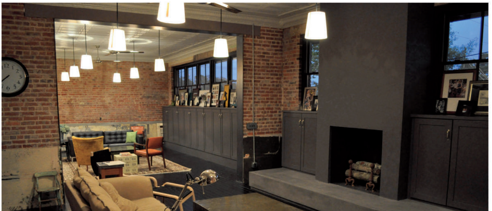
Cutting large openings in the thick brick interior walls helped create an open flow between what used to be four separate commercial spaces.
